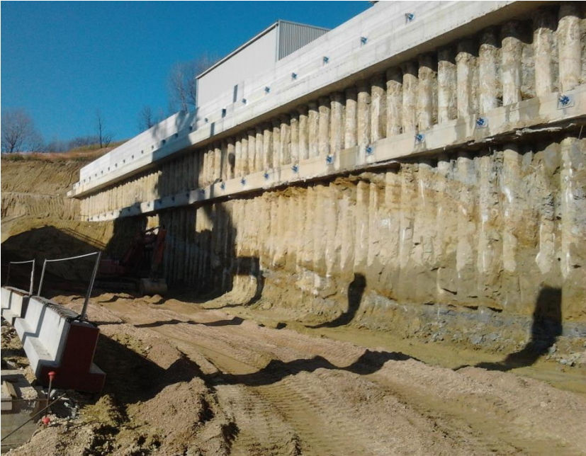
Propped retaining walls
