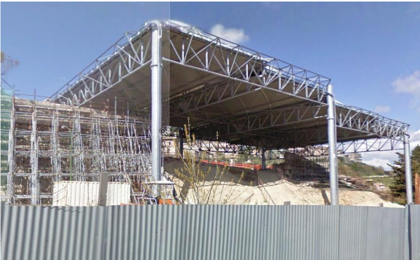
Amelia ancient walls- temporary cover after collapse in 2005
